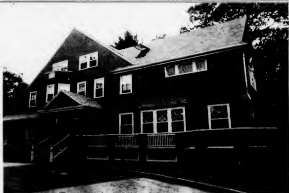
Quinby House, formerly the Psi Upsilon house, recently underwent a $1.5 million renovation. (Gajan Sivakumaran/Bowdoin Orient)
